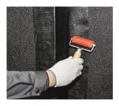
Do not forget to thoroughly flatten and pressure every reinforcement element with a silicone roller.
