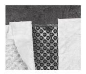
Remove the upper protective film of the sealant tape and fix the next roll of the profiled membrane at the basement level with overlapping width of **4-6 studs**.
