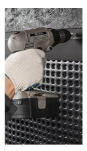
Cover the upper edge of the fixed profiled HDPE membrane with an edge profile.
