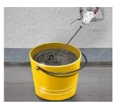
Prepare the mix for installation of fillet (cove), by using mechanical stirring means. It is forbidden to prepare the mix manually.
