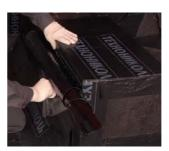
In this case, one should cut the material into shorter segments and first install the material on the lower part of the foundation on its' entire perimeter.
