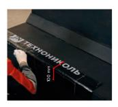
The places of transition from the vertical to the horizontal surface are reinforced with overlaps of **100 mm** on both sides from the bend line.
