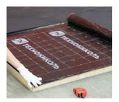
Before the installation of the waterproofing membrane onto horizontal surfaces, measure, cut and align it on place by ensuring the demanded width of overlapping on the longitudinal and transversal edges.
