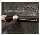
At first, carefully cut and remove the protective film in 100-150 mm from the beginning of the roll and attach the material at the top. Then install the main part of the roll by gradual removing the protective film, unrolling the membrane and smoothing it on the surface.
