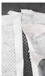
In the place of junction of two rolls of the profiled membrane, provide an overlapping of the free edge of geotextile onto the contiguous roll.
