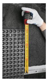
PLANTER standard profiled HDPE membrane is fixed at the basement level with a distance of **200-300 mm** from the waterproofing membrane.
