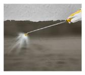
Ensure moisturizing of the laid material (pouring with water, wet bagging, etc.) during the necessary time (indicated by the producer of specific material and usually making 2-3 days under the temperature of +20 °C).
