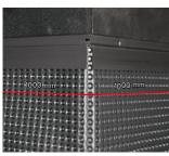
Cover the external corners with whole rolls so that there should be a strip at least 1 m wide in both directions from the corner.
