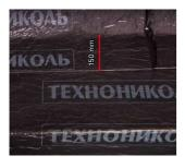
Transversal overlaps of **150 mm** are arranged on the horizontal part of the foundation slab.
