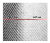
Cover the external and internal corners with whole rolls so that there should be a strip at least **1 m** wide in both directions from the corner.
