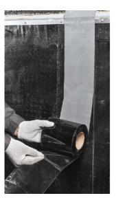
Seal the places of the future vertical junction of contiguous rolls with double-sided self-adhesive sealant tape NICOBAND DUO **150 mm** wide. Do it by removing the protective film carefully from the lower self-adhesive surface of the tape, gradually unwinding the roll from top to bottom and smoothing it by hand.
