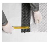
The overlapping of contiguous rolls of the profiled membrane should make 70-100 mm.
