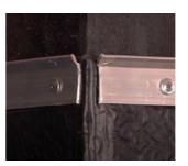
The fastening span is **200 mm**. In the areas of external and internal corners of the construction, as well as while fixing the edge of the metal strip, the fastening span should be reduced to **50 mm**.
