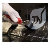
Never forget to thoroughly flatten and pressure every reinforcement element with a silicone roller
