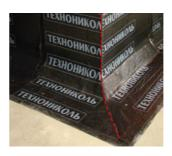
While arranging the external corner, the main waterproofing membrane is installed without overlaps in a toe-to-toe manner.
