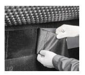
In the places of intermediate fixing of wall drainage at height, remove the upper protective film of NICOBAND DUO and continue unwinding the roll downwards.
