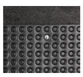
Fix the profiled HDPE membrane with conic studs towards the enclosing structure by means of concrete nails or self-tapping screws with clamping washers.
