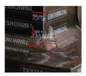
For that, one should prepare patches, similar to those mentioned see in section 4.3. In this case, however, each patch should overlap both sides from the corner axis for **150 mm**, while overlapping the lower element for **100 mm**.
