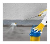
Carefully spill the surface with water until full saturation.
