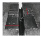
Reinforce the expansion joint area with patches made from the self-adhesive polymerbitumen membrane before installing the main waterproofing layer. The expansion joint with a compensating loop should look as shown in the picture. Each element should overlap both sides from the expansion joint for 100 mm, while overlapping the lower element for 150 mm.
