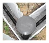
Connect the wall drainage to the pipe drains installed around the perimeter of the structure, arrange the drain fills. Install the inspection and drop wells according to the design.
