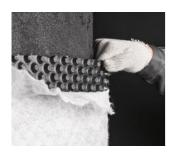
While protecting the external corners with PLANTER standard and PLANTER geo, it is necessary to keep the profiled membrane edge parallel to the corner of the structure. For this purpose, stretch the upper edge of the membrane and only after that fix it to the base. Otherwise, there will be warping of the profiled membrane.
