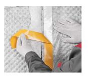
Seal the place of junction of two geotextile sheets with double-sided self-adhesive sealant tape NICOBAND DUO 75 mm wide or regular doublesided adhesive tape. Remove the upper protective film of the sealant tape.
