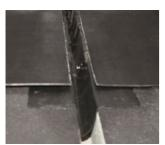
Proceed with the regular installation of the main self-adhesive waterproofing membrane while not overlapping the expansion joint itself.
