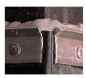
In the places of interruption of the edge strip, apply the sealant in a continuous layer.
