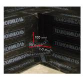
Then additional reinforcement elements are installed from the bottom upwards overlapping both sides from the corner axis for **150 mm** and the lower element for **100 mm**.
