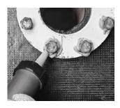
Also treat the anchor bolts with polyurethane sealant before tightening them.
