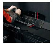
The places of transition from the horizontal to the vertical surface are reinforced for the height of the fillet plus overlaps of **100 mm** on both sides from the fillet.
