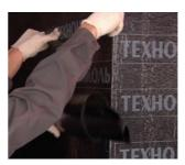
Proceed with the installation of the main waterproofing membrane on the vertical walling. Make the holes for anchor bolts in the main waterproofing membrane only after its' installation.
