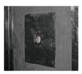
Reinforce the penetration with the patch made from the self-adhesive polymer-bitumen membrane before installing the main waterproofing layer on the vertical walling. Do not forget to thoroughly flatten and pressure the reinforcement element with a silicone roller to avoid the formation of air bubbles and creases.
