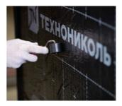
Always use silicone roller to ensure reliable adhesion of the material to the surface and avoid the formation of air bubbles and creases, which can worsen the waterproofing properties.
