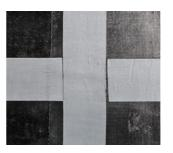
If the intermediate fixing of the wall drainage at height is required, attach NICOBAND DUO tape **150 mm** wide in the respective places.
