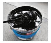
Carefully mix the primer by a low-speed drill with the special nozzle.
