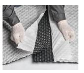
Prepare the rolls of PLANTER geo profiled HDPE membrane for installation. For this purpose, take off the geotextile carefully from the edges of contiguous rolls for a width of 4-6 studs.
