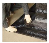
Then additional reinforcement elements made from the main non-reinforced self-adhesive waterproofing membrane are installed on all joints of the corner starting from the bottom.
