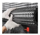
Unwind smoothly the roll of profiled membrane fixed at the basement level in downward direction.
