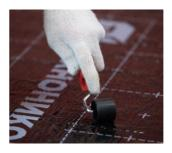
Make sure that no cavities or air bubbles occur between the material and the base. For that, use the silicon roller during installation.
