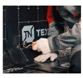
For better adhesion, clean the overlap zone from dirt and dust with the clean and dry cloth just before the formation of transversal or longitudinal overlap and press it with the roller after the installation of the material.
