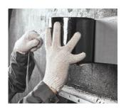
The wall drainage can be fixed at the basement level with double-sided self-adhesive sealant tape NICOBAND DUO 150 mm wide. For this purpose, stick the tape at the level of 200-300 mm above the waterproofing membrane.
