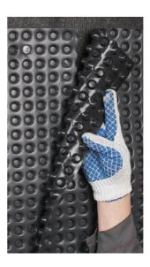
The lateral overlapping of adjacent rolls should make at least **4 studs**.
