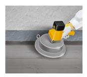
Clean the place to arrange the fillet (cove) from cement slurry, dust and dirt.
