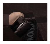
Reinforce the free area of the corner with another small patch overlapping the underlying element.
