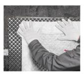
Fix PLANTER geo profiled HDPE membrane with doublesided self-adhesive sealant tape NICOBAND DUO at the basement level.
