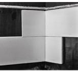
Start installation of XPS slabs from the corners. In order to avoid formation of thermal bridges, install the slabs of adjacent rows with spacing of joints of half the slab size.
