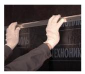
One should finish the installation of the self-adhesive waterproofing membrane on a vertical surface with mechanical fixation. To do so, fix the upper edge of the waterproofing membrane to the structure at the basement level with profiled metal edge strips along the entire perimeter of the construction.
