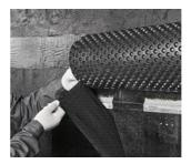
After that, wind up the roll of the profiled membrane upwards. In the place of vertical junction of contiguous rolls, remove the upper film of NICOBAND DUO and gradually unwind the wall drainage roll downwards.
