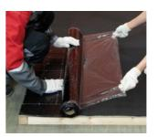
Then install the remaining part of the material by gradual removing the film and rolling out the membrane. Avoid shifting the roll from its' desired position.
