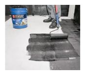
Apply the primer manually onto the cleaned surface with brushes, sweepers or paint rollers.
