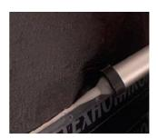
Fill in the space between the wall and the folded flange of the edge strip with a polyurethane sealant.
