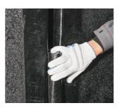
Form the compensating loop by using the main waterproofing membrane wound into the roll.
