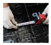
The longitudinal overlap should be minimum 100 mm, transversal — not less than 150 mm. Transversal overlaps of adjacent rows should be displaced for at least 500 mm.
