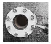
Fix the clamping plate with anchor bolts. Before definitive tightening of bolts, apply a polyurethane sealant to the place of adjunction of the clamping plate to the waterproofing membrane.
