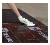
For better adhesion, it is recommended to clean the overlap zone from dust just before the installation of the following roll and press the material with the roller after its' attachment.
