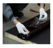
Start installing the first row of the membrane. Carefully cut and remove the protective film in **100-150 mm** from the beginning of the roll.
