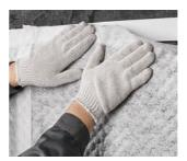
Stick the upper free part of geotextile sheet to double-sided self-adhesive sealant tape NICOBAND DUO **75 mm** wide or regular double-sided adhesive tape.
