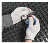
If necessary, perform intermediate fixing of the profiled membrane at its' height by using a mechanical fixture attached directly to the waterproofing membrane. To install the fixture, it is necessary to remove the protective film on its' platform and stick the fixture to the waterproofing membrane.
