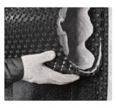
Unwind the roll downwards by carefully pressing the places of overlapping and intermediate fixing.
