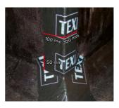
Then reinforce the vertical part of the external corner with **50 mm** overlap on the lower element and **100 mm** overlaps on both sides from the corner axis.
