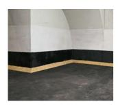
Allow the treated surface to stand until the full drying of the primer. The primer drying time depends on its' type and environmental conditions during the work.
