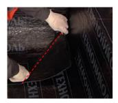
Waterproofing of the internal corner is arranged similarly. The main waterproofing membrane is installed without overlaps.
