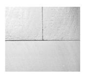
Then continue with installation of entire slabs. The spacing of joints in adjacent rows will appear at the middle of the slab.
