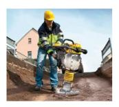
The backfilling is performed by layers with careful ramming of each layer up to the soil consistency values specified in the design.
