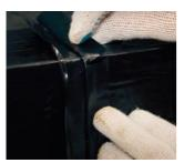
The next reinforcement element made from the main non-reinforced self-adhesive polymer-bitumen membrane is installed toe-to-toe to the previous one without any overlap.
