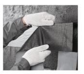
Start fixing the rolls of profiled membrane from the upper point (basement level). At first, remove the upper protective film of NICOBAND DUO.
