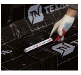
The longitudinal overlaps should be minimum **100 mm**.
