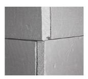
Change the direction of XPS slabs connection in adjacent rows in corner area.
