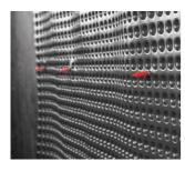
Pierce through the roll of profiled membrane with the tip of the fixture.
