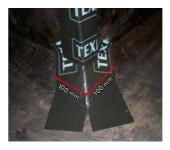
The reinforcement of the external corner is performed in two steps. At first, one should reinforce the lower part of the corner adjacent to the horizontal surface. For this, make a patch from the main waterproofing membrane with special cutouts so that the element can be installed without waves and folds. The element should overlap both sides from the corner axis for **100 mm**.
