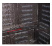
The longitudinal overlaps of upper and lower segments of the vertical membrane should be displaced for at least **300 mm**.
