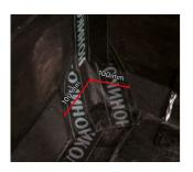
The reinforcement of the internal corner is done in a similar manner. Start with the installation of the patch with cutouts in the lower part of the corner adjacent to the horizontal surface. The element should overlap both sides from the corner axis for **100 mm**.
