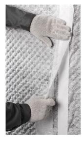
Stick the geotextile sheet of the contiguous roll to the sealant tape.
