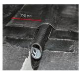
Finally, install additional reinforcement elements made from the main non-reinforced self-adhesive waterproofing membrane on top of the formed compensating loop. Each additional reinforcement element should overlap both sides from the expansion joint for 250 mm, while overlapping the lower element for 150 mm.
