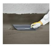
Apply the prepared mix onto the surface, by forming a fillet (100×100 mm size) or a cove (R=100 mm).
