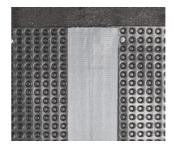
The joint sealing is necessary to avoid outside elements (ground, waste etc.) in the profiled membrane in the course of further operations.
