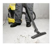
Before applying the primer, clean the concrete surface from dirt and dust. In case of using a compressor for this purpose, it is necessary to ensure that it is equipped with a moisture and oil separator.
