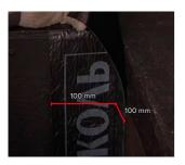
Then reinforce the vertical part of the internal corner with **50 mm** overlap on the lower element and **100 mm** overlaps on both sides from the corner axis.
