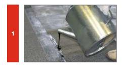
The surface must be cleaned of dust, debris, grease, leaves and other items that can reduce the adhesion of the waterproofing material. In addition, the surface should be aligned, dry and should not have gaps and cracks or other irregularities.
