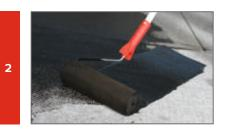
Surface must be properly prepared before installation of waterproofing material. For this purpose, it is recommended to use bitumen primer TECHNONICOL No.01 or No.04, which improves the adhesion of roll material.
