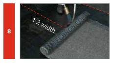
Cap sheet membrane should be positioned at a distance of min. 300 mm from overlaps of underlay membrane. Usually it is moved at a distance of 500 mm (50% of roll width).
