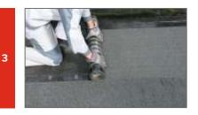
Before installation, the material has to be rolled out and aligned on a place where it is going to be installed. Roofer has to straighten all rolls and pay attention to lapping of adjacent membranes. The distance between different end laps of rolls should be at least 500 mm. Then the material has to be re-rolled tightly from both sides towards the center avoiding position changes of the membrane. Prepared material has to be torched-on from the center of the roll to both sides.
