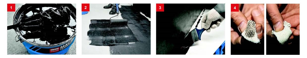
Carefully mix the primer by a lowspeed drill with the special nozzle. Apply the primer manually onto the cleaned surface with brushes, sweepers or paint rollers. Corners and other hard-to-reach spots must be daubed with a hard-bristle brush. Allow the treated surface to stand until the full drying of the primer. It is possible to check whether the primer has dried by pressing a dabber to it: there should be no bitumen traces on the dabber pressed to the dried primer.
