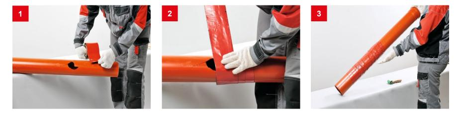
To repair the damage on pipes, the tape is wound spirally (with an overlap on the previous turn). Self-adhesive sealant tape NICOBAND gives an opportunity to feel professional in construction and repair.
