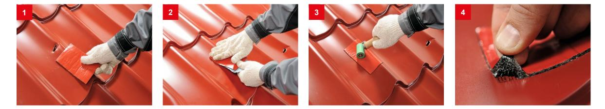
Self-adhesive sealant tape NICOBAND is suitable for repair of any roof from natural or metal colors, which allows to easily find shingles, bitumen shingles, bitumen or seam roofing.
