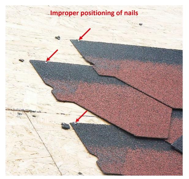
Application failure due to the wrong nails type (nail head should be not less than 9 mm in diameter)
